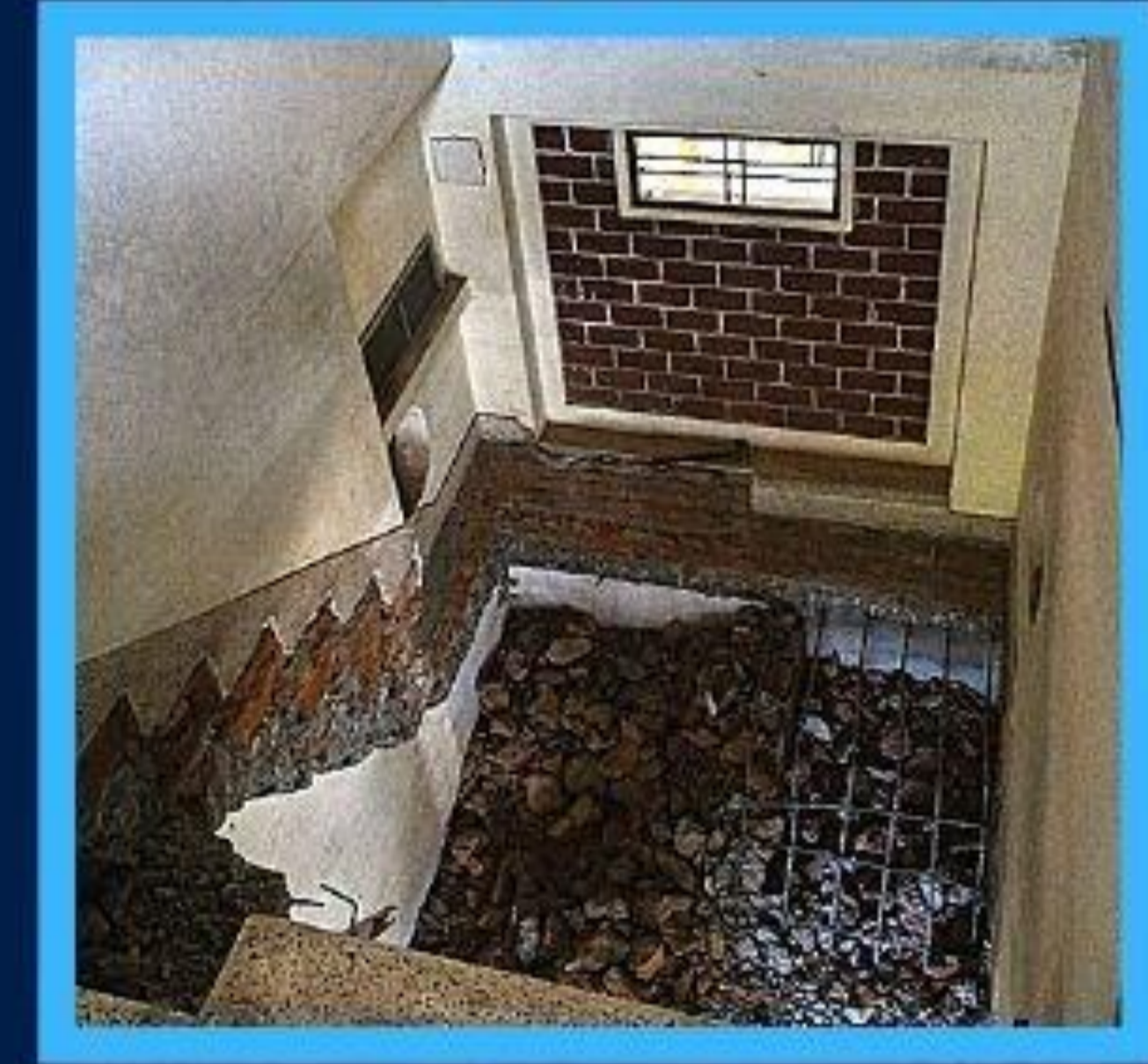
STAIR REALIGNING
